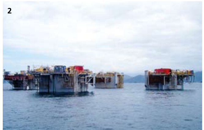
To achieve the required mating draft, the hull was ballasted down
