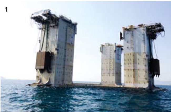
FloaTEC towed the hull from the BrasFELS yard to a deepwater mating hole near Angra dos Reis
